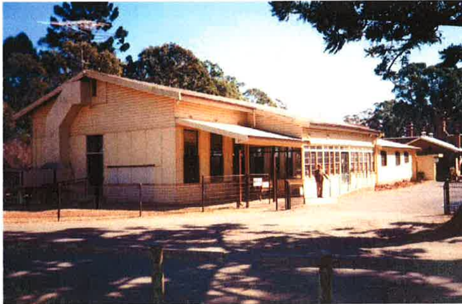
Figure 28 The Original Parry Ward taken in 1994 just prior to its demolition for the construction of Parry House.
