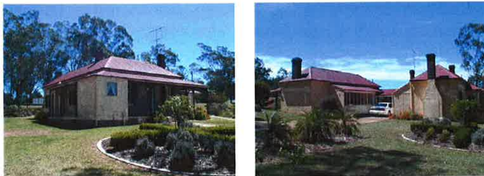
Figure 33 - Grasmere Villa, showing its east (main entrance) and west (service courtyard) elevations.
