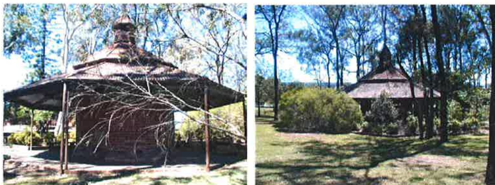
Figure 30 - Original mortuary, extensively modified as an entertaining area
