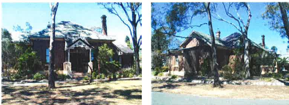
Figure 31 – The Masonic Cottage Hospital, west elevation showing the main entrance and the northwest corner.
